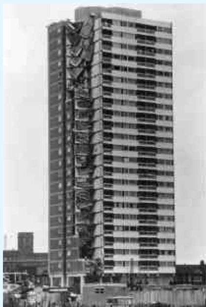
Figure 6 Ronan Point following collapse
