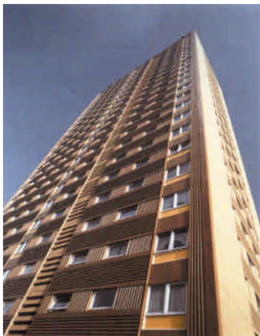
Figure 13 One of many different approaches to over cladding in this case to a Reema block. Timber battens carrying colour coated aluminium sheets. A combination of vertical and horizontal ribbing. Panels fixed back through a neoprene gasket. Insulation: 25 mm of polystyrene board
