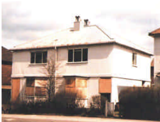
Figure 1 Telford steel framed house -1920s - this was one of the steel clad systems
