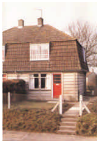
Figure 2 Cornish Unit Type 1 – one of the many types of pre-cast reinforced concrete houses
