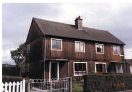
Figure 3 Swedish Timber (As a result of a wartime purchasing commission visit to Sweden in 1945 Swedish Timber dwellings were imported in pre-fabricated sections for erection to English and Scottish designs)
