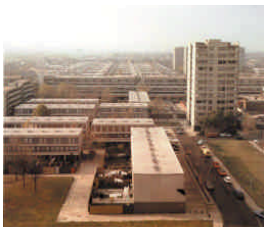
Figure 5 Large panel System – Balancy General view of estate
