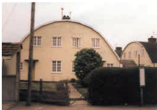
Figure 9 Nissen-Petren steel framed house - The range of systems and construction techniques used has been extremely varied and includes some unusual-looking house types
