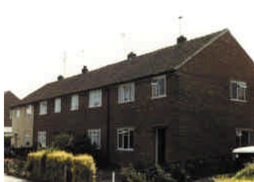
Figure 10 Spooner timber framed house – looks traditional
